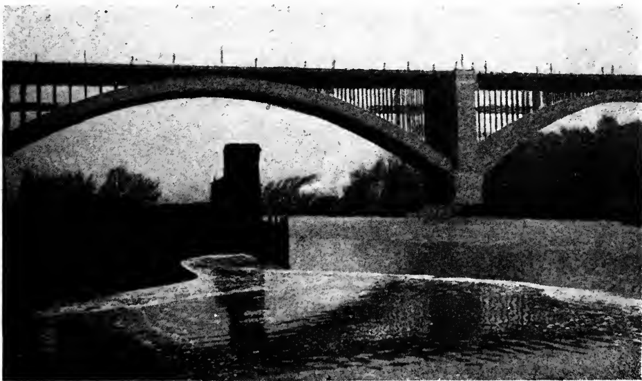
WASHINGTON BRIDGE, HARLEM RIVER.
